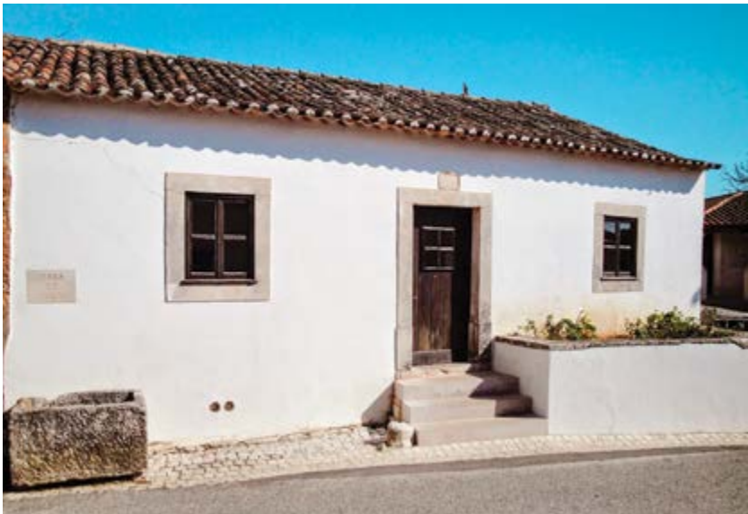
The family home of Lucia after renovation
